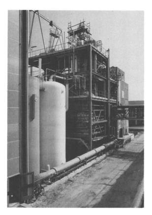
Figure 1. A 200-m³ PVC reactor installed at Chemische Werke Hüls with a capacity of 30,000 to 50,000 tons/year of PVC grade suspension or emulsion
